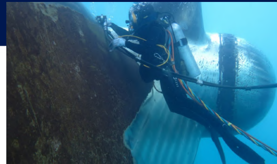
Underwater propeller polishing
